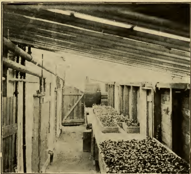
14.—Interior of shed shown in Figure 13. Propagating bench on the right, supply pipes (two-inch) on the left, shed eight feet wide
